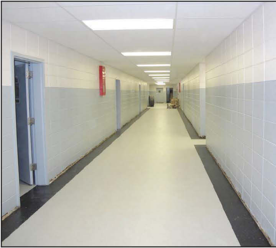
The GCTC office, halls and classrooms received a makeover during the summer providing a bright, inviting environment for students. New lighting, dropped ceilings and new tile and color scheme will enhance the students experience at GCTC.
